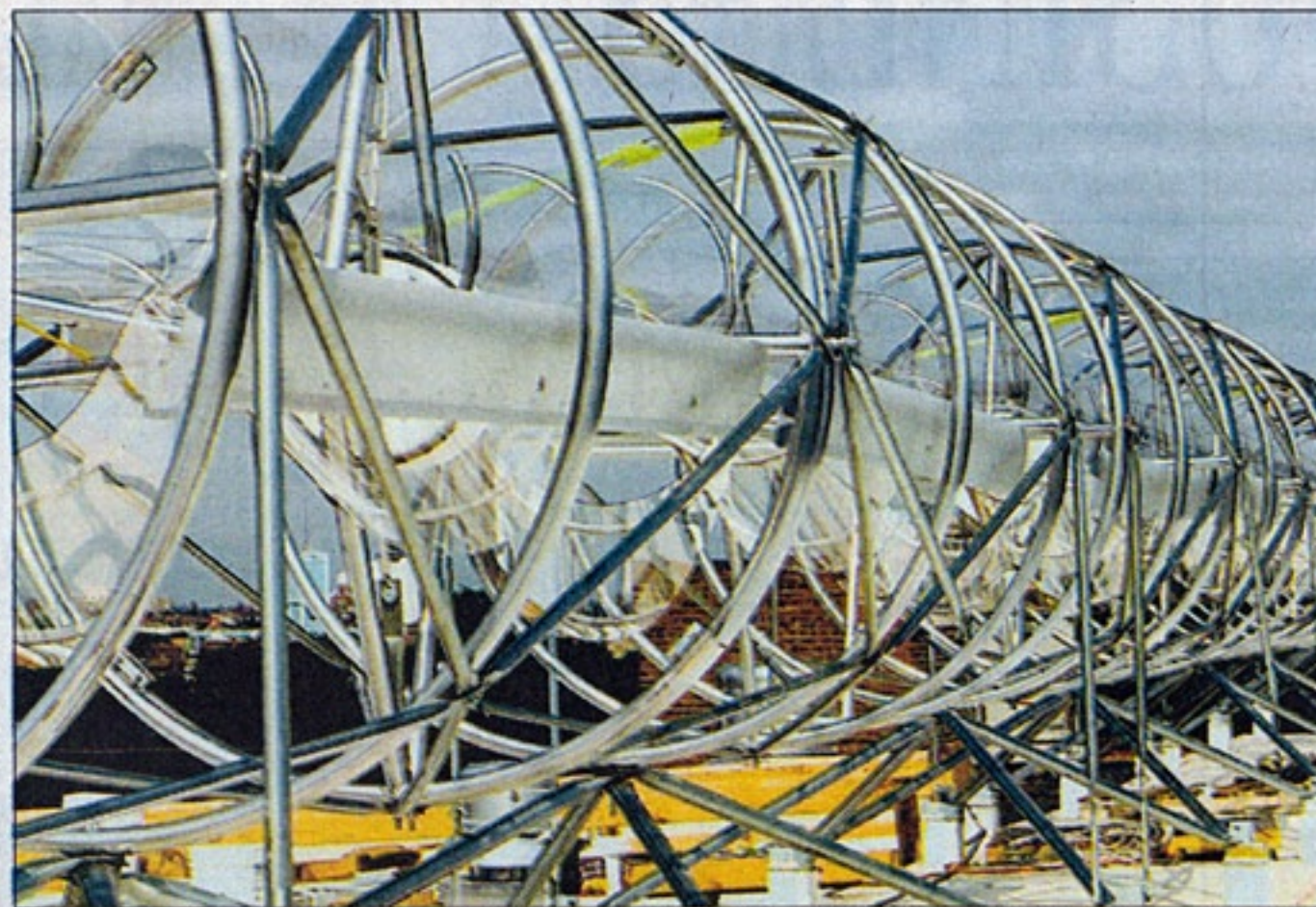
Rooftop wind turbines, which generate energy for use in commercial and residential buildings. Pfister Energy of Paterson expects to install more than a dozen turbines this year on top of a clothing importer's building in Fort Lee. The 10-foot-high turbines would be visible to drivers on the George Washington Bridge.
