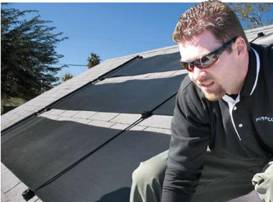
Solar pool heating installers from Fafco Inc. install three polypropylene panels on a home in California. Water circulates through these panels, is heated, and gets pumped back into the pool.
