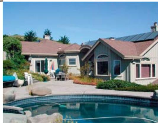
**Residential solar pool system by Solar Depot using the polypropylene copolymer panels.**
