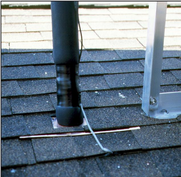
Completed installation of roof flashing with pipe insulation.
