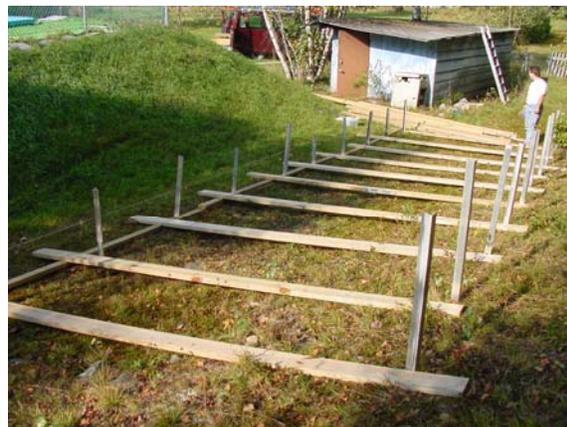
Shown above are the posts for an eight panel system all in place. The six inch rafters are ready to be bolted to the supporting posts. In this application the panels are 12' in length, therefore the rows of posts are 10' apart.
