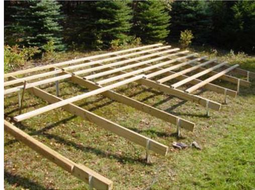
After all the rafters are bolted to the posts the decking 2 x 4's can be fastened to the rafters. The spacing for the decking is approximately 13 to 14 inches on center depending upon panel length. The overall spacing on the top and bottom planks are one inch less than the panel length.
